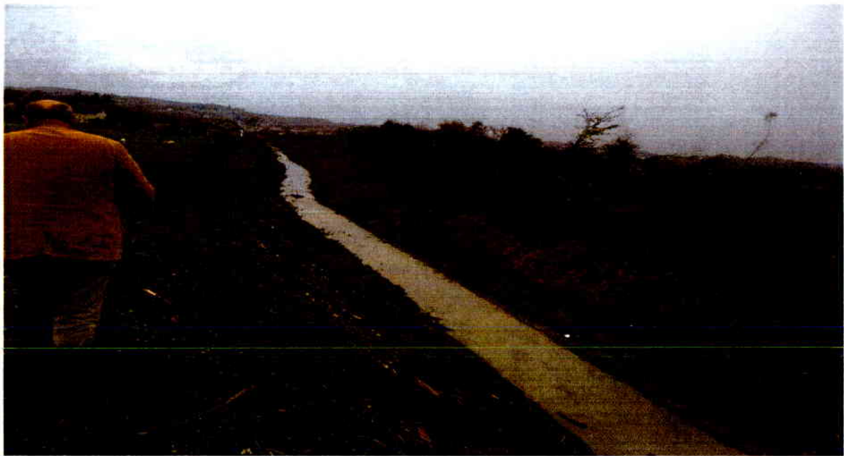
Photo: result of construction works on cleaning and regulation of Mahovljanska river
