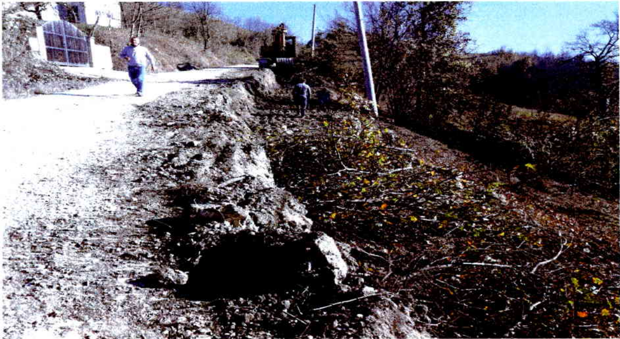
Photo: Construction works on rehabilitation of landslide in Maglaj
